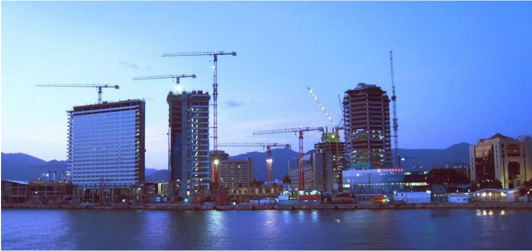
The Port of Spain International Waterfront Centre
